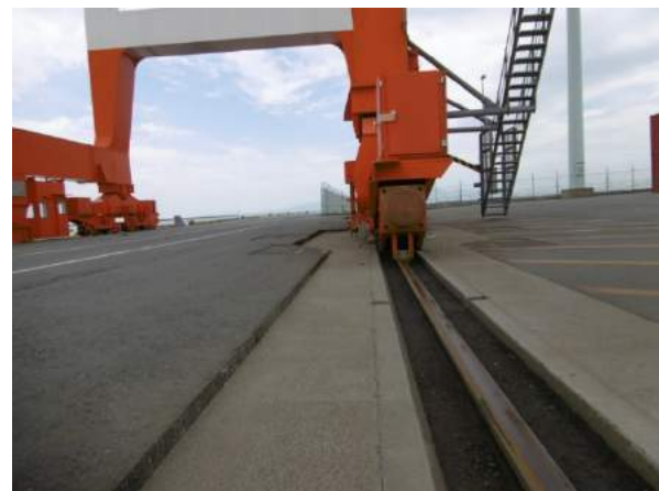
Photo 1: Slight damage to a quay wall at the Port of Kumamoto
